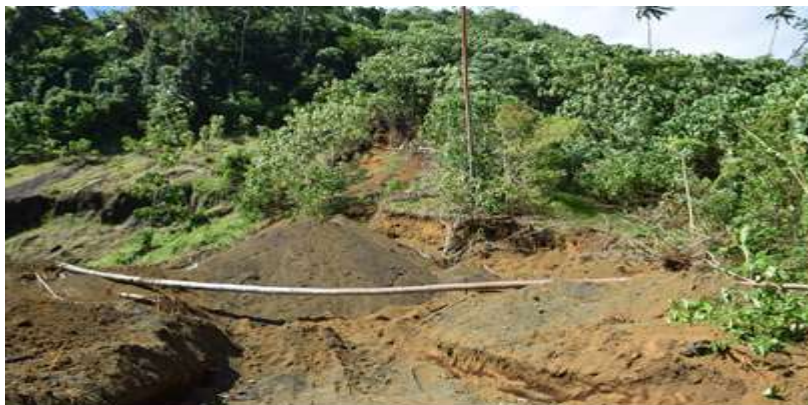
Extractive sand mining on the side of the Tafua crater causing soil erosion and the high risk of a landslide during extreme heavy rainfall. Photo credit: MNRE-PUMA. 2017
