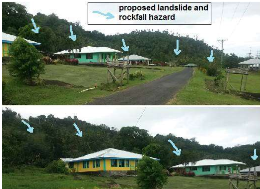
Unstable crater wall of the Tafu-a-savaii Volcano, this has high risk of triggering a landslide and rockfall (blue arrows) in the area. Photo credit: Aleni Fepuleai, 2017
