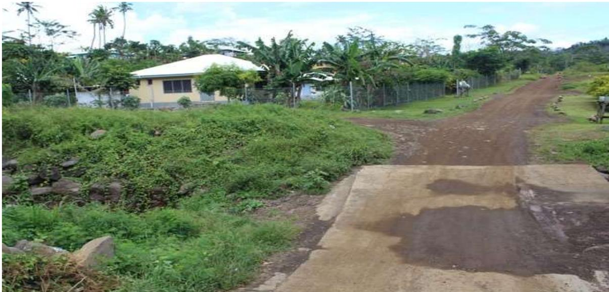
Ford at Moamoa-fou towards Catholic Resettlement Area, when it is heavy rain and flooding it will stop vehicles from crossing and can isolate families on the other side of the ford with no access to cross if there is an emergency. Long term solution is replace ford with a bridge
