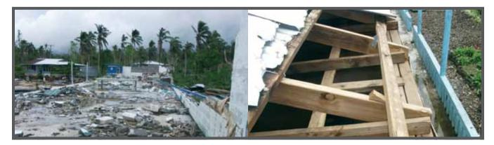
Photos Left: Salamumu Primary School, total rebuild required from foundations up. Right: Faleseela Primary School, Strengthening required for roof structure tie downs. Courtesy of GoS/PDNA Assessment team.
